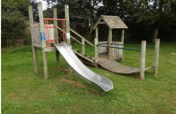
**Finding:** There is/are finger entrapment/s in the structure and the item fails to meet the requirements of BS EN 1176 Part 1 4.2.7.6 Entrapment of fingers
