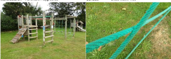
Finding: The ropes/nets are worn/damaged in places
