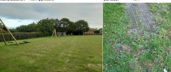
Finding: The grass mats are silted up and the soil is compacted; this may have an effect on the impact absorbing ensure the correct surface qualities are maintained for the properties of the surface
