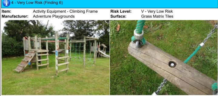
**Finding:** There is/are bolt cap covers missing or damaged on the item
