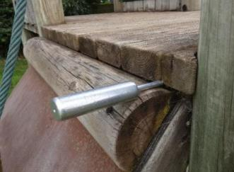
**Finding:** There is/are finger entrapment/s in the structure and the item fails to meet the requirements of BS EN 1176 Part 1 4.2.7.6 Entrapment of fingers
