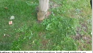
Action: Monitor for any deterioration (rot) and replace as required
